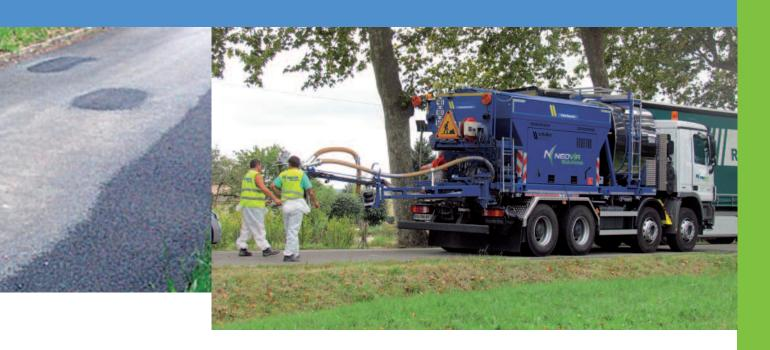
The technique of the Sprayed asphalt to bitumen emulsion guarantees, in a single passage of the workshop, a durable repair of these types of degradation.
